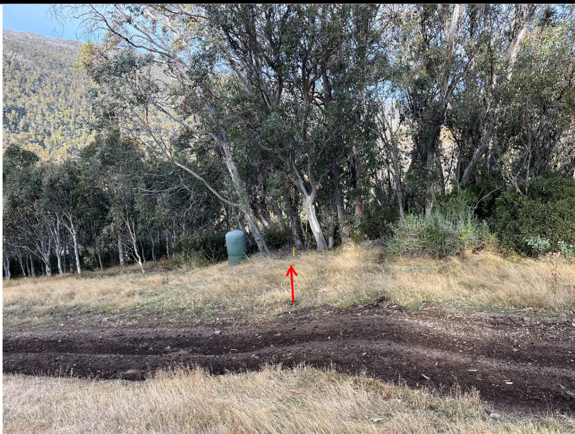
New fan pit, TT10 fan gun and lateral from snowmaking mains.
